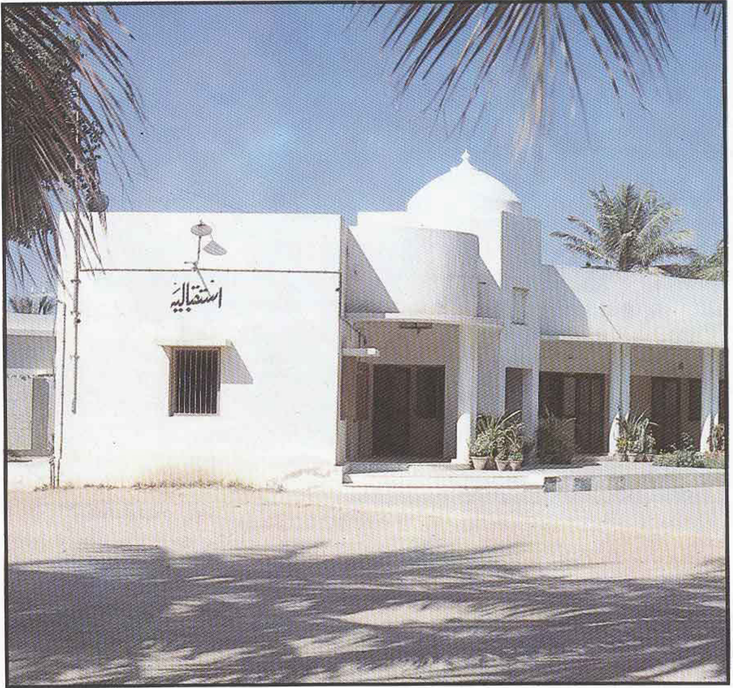
Reception, Telephone Switchboard and other Managerial Offices
